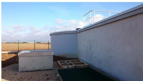
Figure 8. Installations de surface F2
